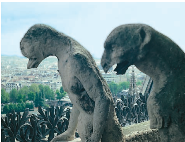
(A) Weathering is especially obvious on old monuments in Europe. Here, most of the details on the gargoyles of the Notre Dame Cathedral in Paris have been erased by weathering.
